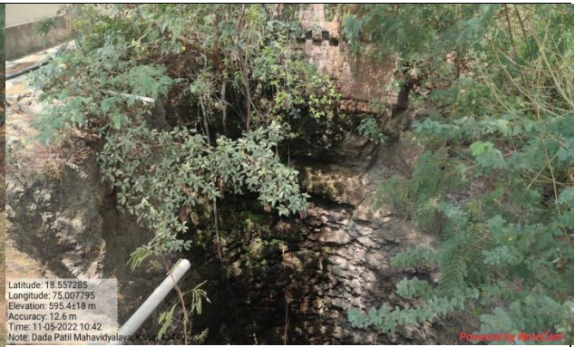
Bore well /Open well recharge
