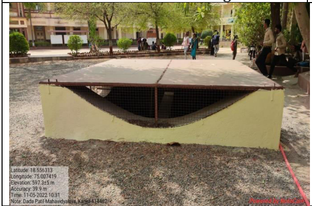
Construction of tanks and bunds
